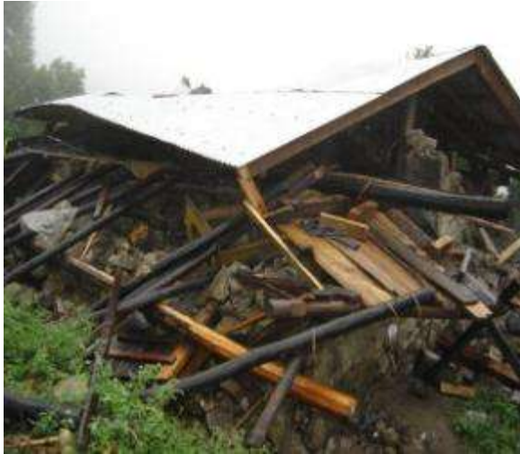
Durung: Total collapse of a house killing one and major cracks to another house
