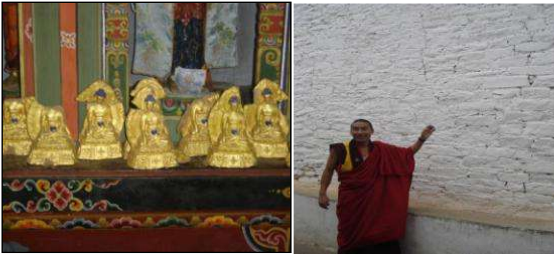
Drametse: Earthquake damage to inner statues as well as exterior Monastery walls
